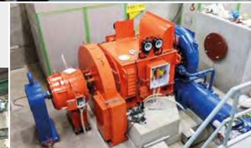
Akinci - I/II, Turkey Type of Turbines: 'PIT' Type – Axial Flow Rated Head: 6.40 m Installed Capacity: 4 x 3,600 kW
