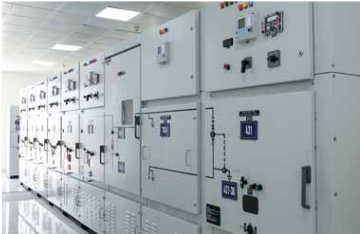
Solar EaSup 1 Switchgear Panels
