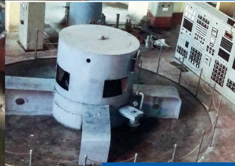
Upper Sindh, Stage II, HEP, India Type of Turbines: Vertical Francis Rated Head: 224.00 m Installed Capacity: 3 x 35,000 kW
