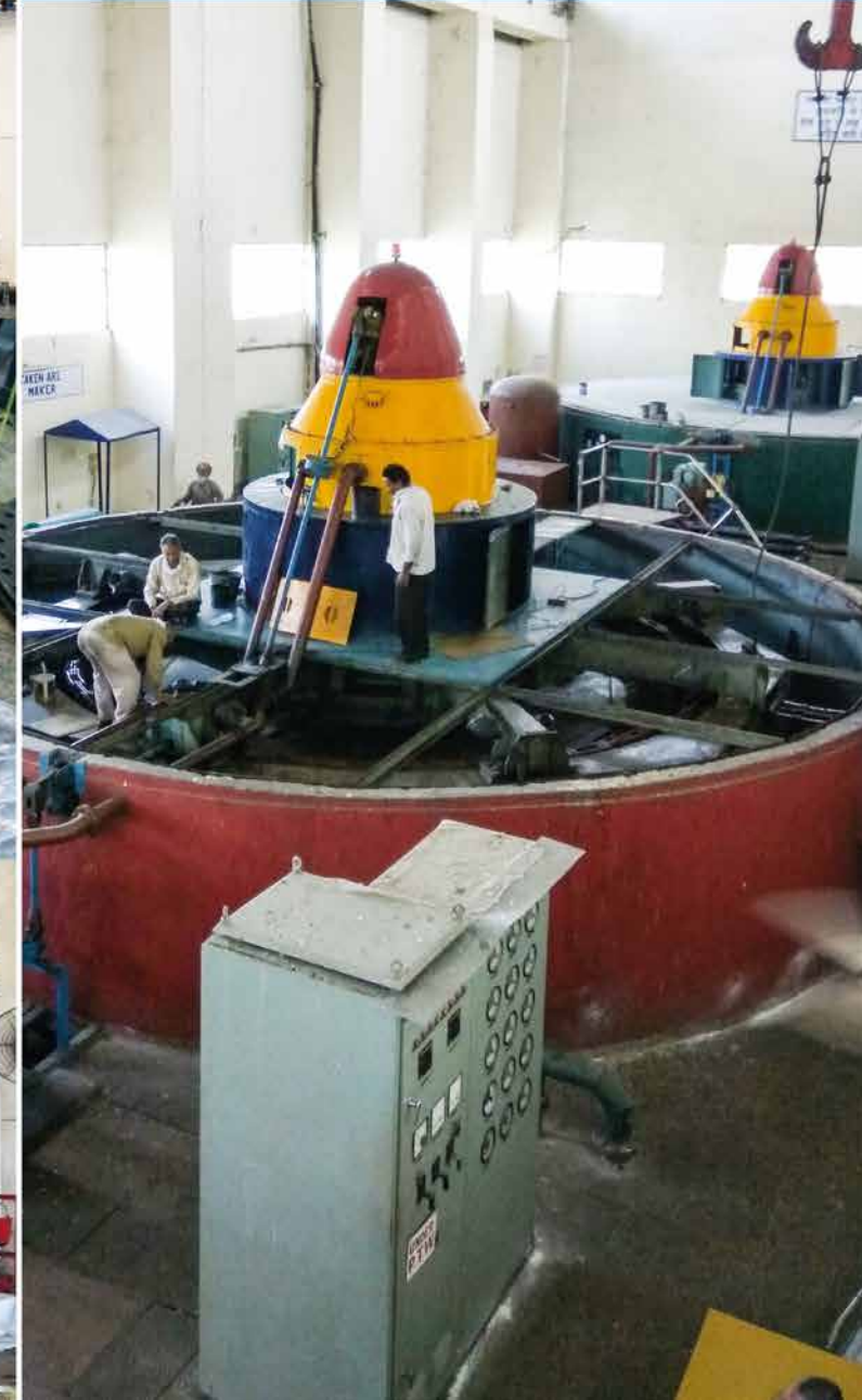
Mukerian, India Type of Turbines: Vertical Full Kaplan Rated Head: 16.80 m & 22.00 m Installed Capacity: 6 x 15,000 kW + 6 x 19,500 kW
