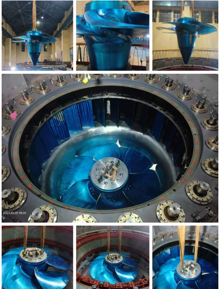
Figure 7: Installation of the new turbine at the plant
