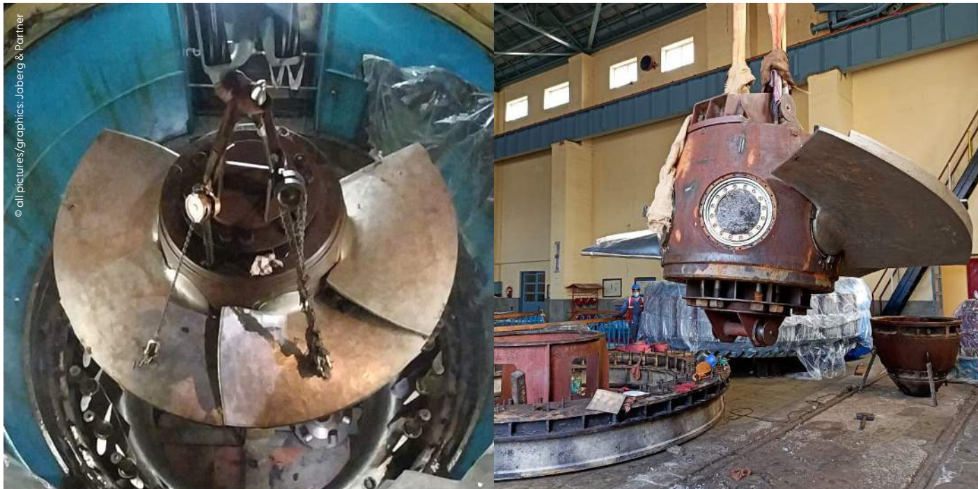
Figure 1: Photographs of the dismantled turbine on site
